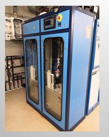
Line 1 AsH3 Line 2 AsH3 Line 3 PH3 incl purifier Line 4 AsH3 Line 5 PH3 Line 6 DEZn Line 7 Cp2Mg / CBr4 1x 4 way Epifold manifold
